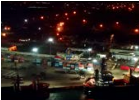
SAGARMALA PROJECTS - PARADIP Container Berth
