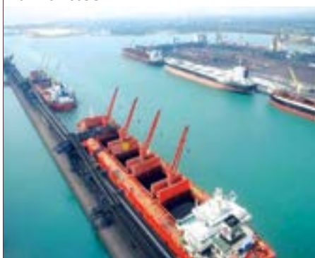
SAGARMALA PROJECTS - PARADIP New Deep Draft Coal Import Berth on BOT basis
